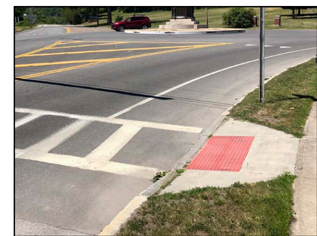
Image E: Example of proposed striping method for existing and new crosswalks along Montcalm Street.
