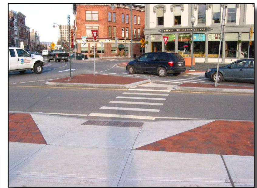
Image A: Example of traffic circle with raised islands and striped crosswalks, helping to bring definition and order to a large roundabout intersection.
