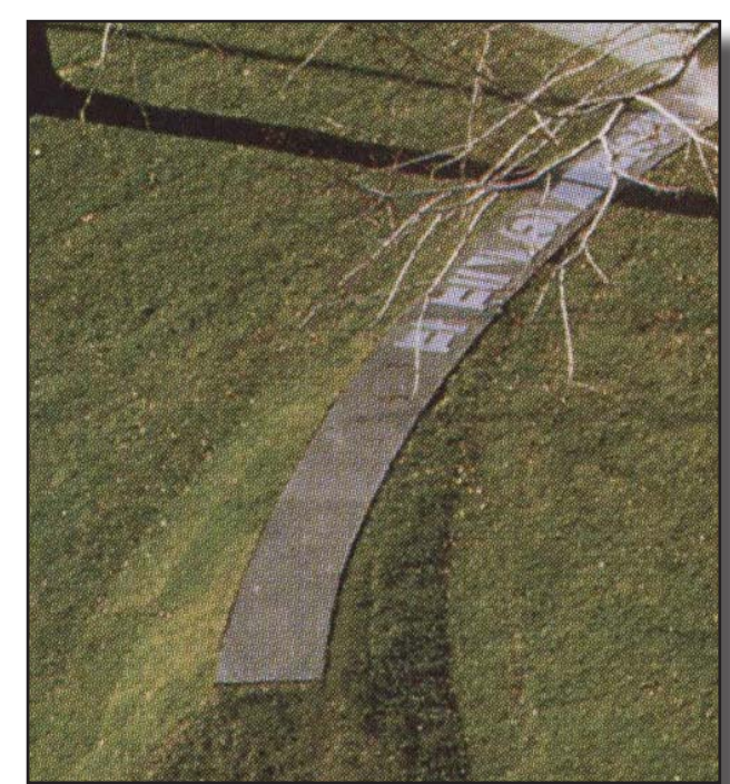
Photograph T: This image shows a turf grass berm that is lower to the ground and would require less fill material.
