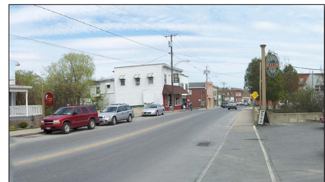
View of Montcalm Street crossing the LaChute River looking east.
